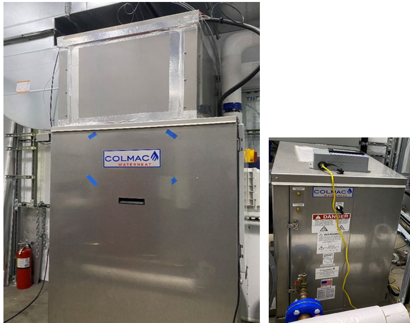
Figure 5. Colmac CxA-15 (left) and Colmac CxV (right) as installed for testing.
