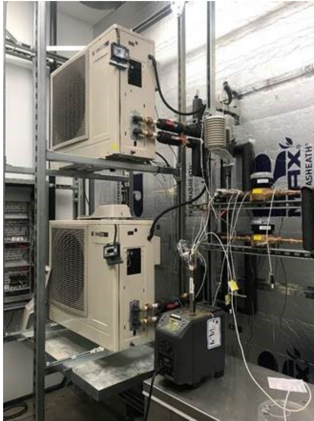
Figure 4. Two Sanden Gen3 units as installed for testing.
