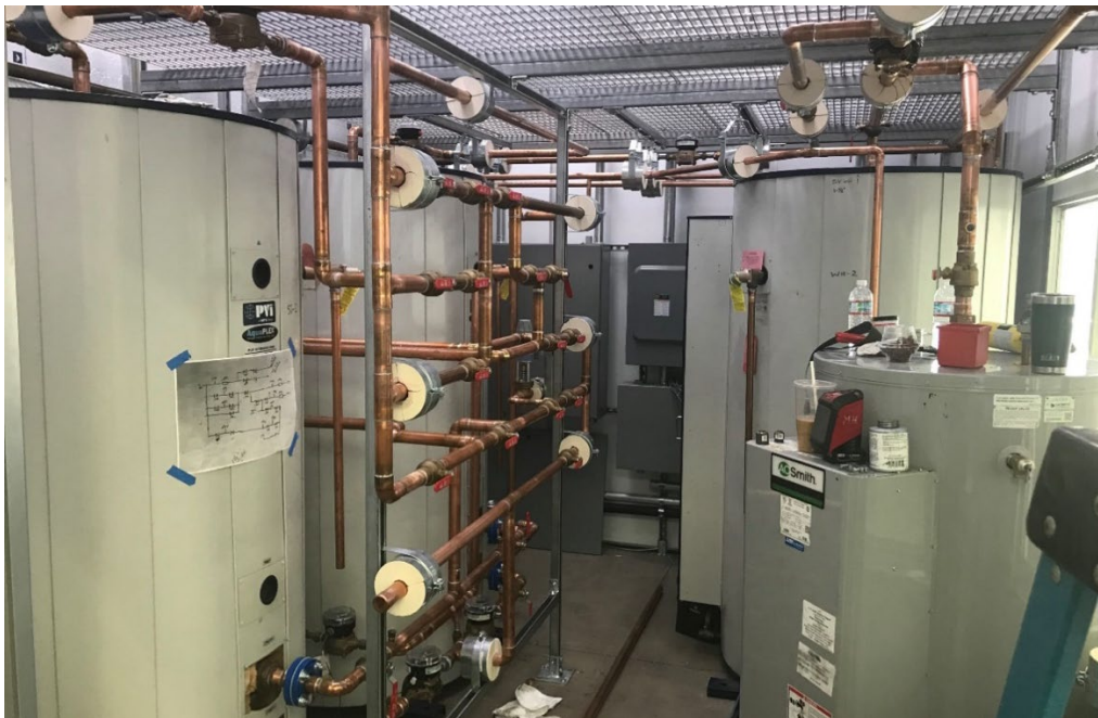
Figure 3. Lab test bed under construction.
