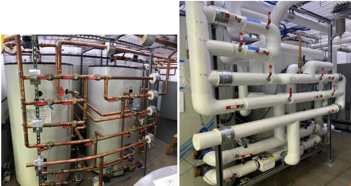
Figure 11. Main valve and configuration switching station before and after insulation was installed.
