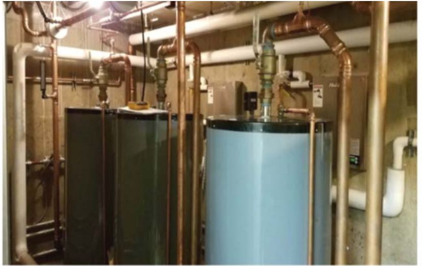
Figure 4. Primary DHW Storage Tanks Before Pipe Insulation (ST1, 2, and 3)
