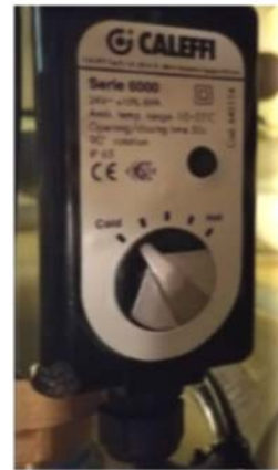
Figure 5. Electronic Mixing Valve and Valve Controller (TMV-1)
