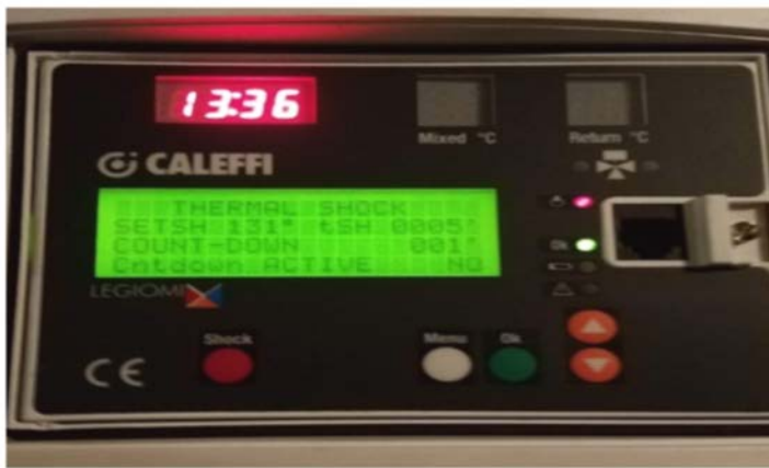
Figure 5. Electronic Mixing Valve and Valve Controller (TMV-1)
