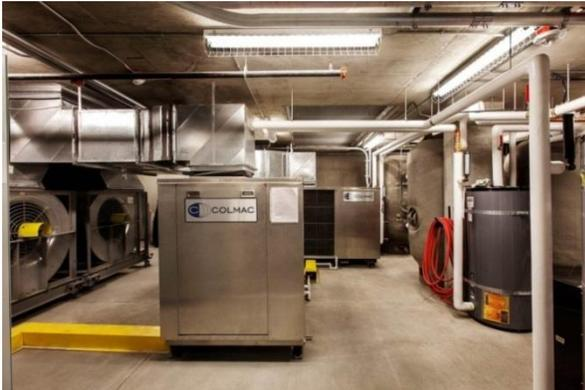
Figure 3: Colmac Industries RCC Equipment
