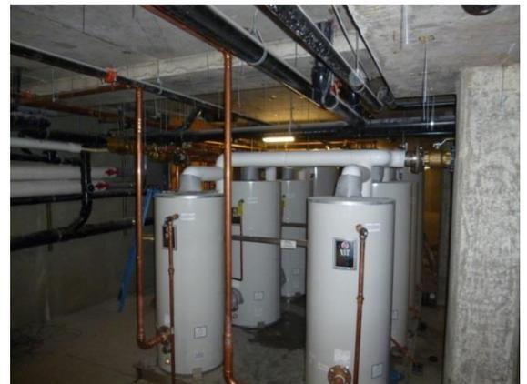
**Figure 7: Domestic Hot Water Storage Tanks in Parking Garage**
