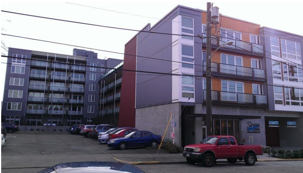
Figure 1: Stream Uptown Apartments – The first RCC Pilot project to be completed in Seattle
