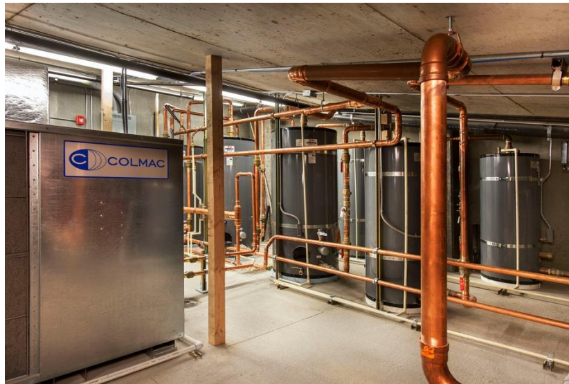
Figure 7: Sunset Electric RCC System During Construction
