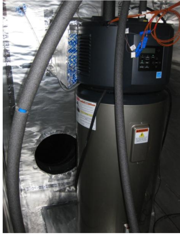
Figure 3. GeoSpring Installed in Test Chamber
