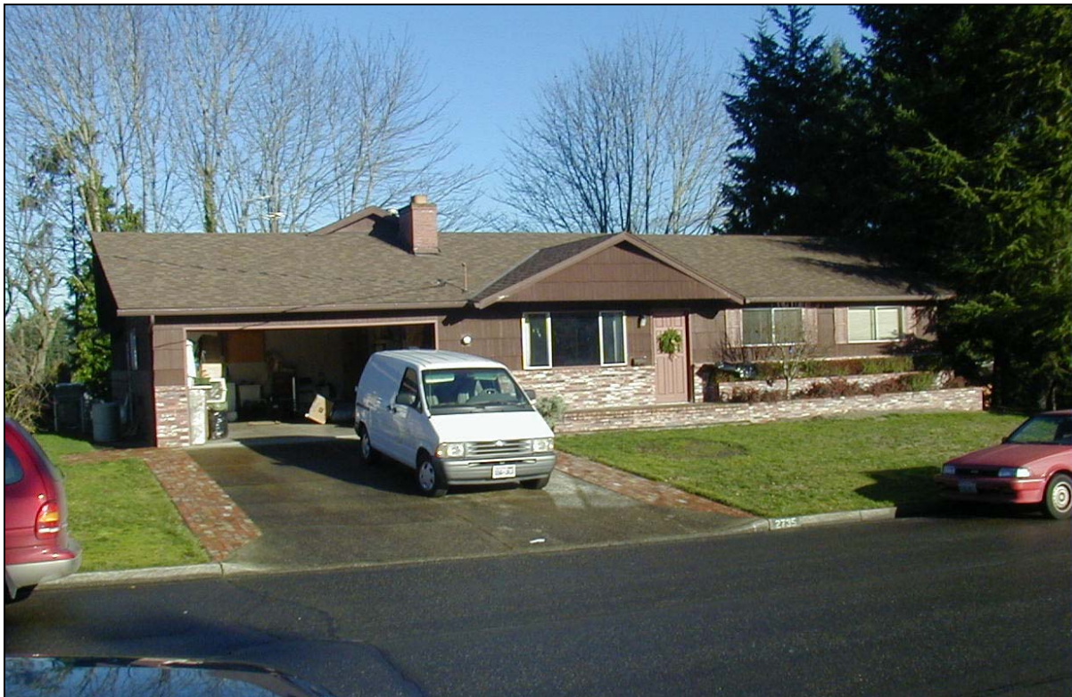
Figure C1. Front view of Site L03.
