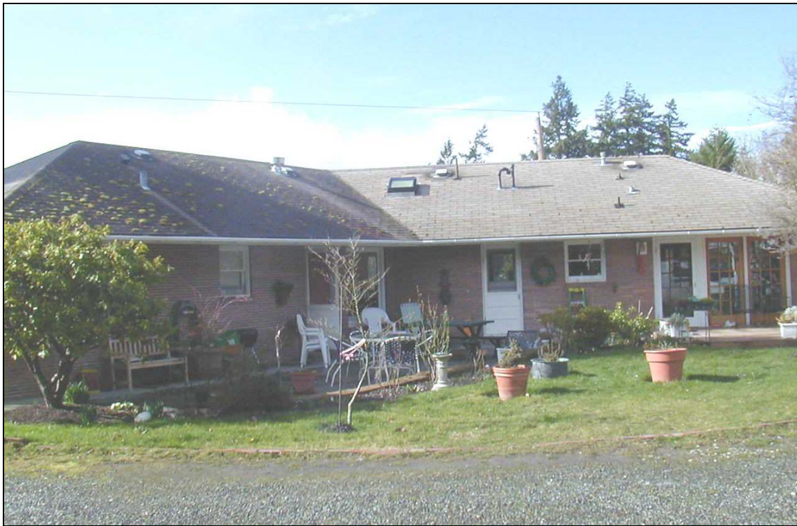
Figure E1. Front view of Site L05.
