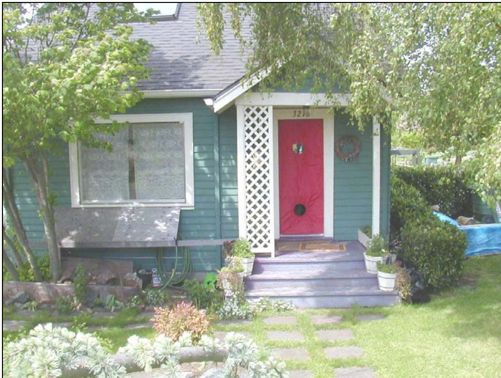
Figure I1. Front view of Site L09.
